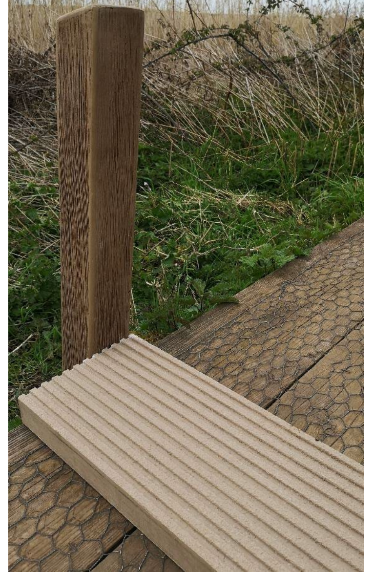
Contrasting wood-effect handrail.
